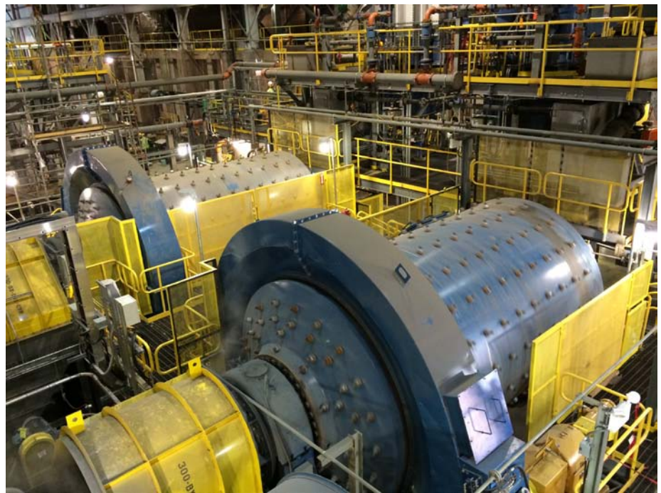
Ball Mills at Eagle Mine's Humboldt Mill
